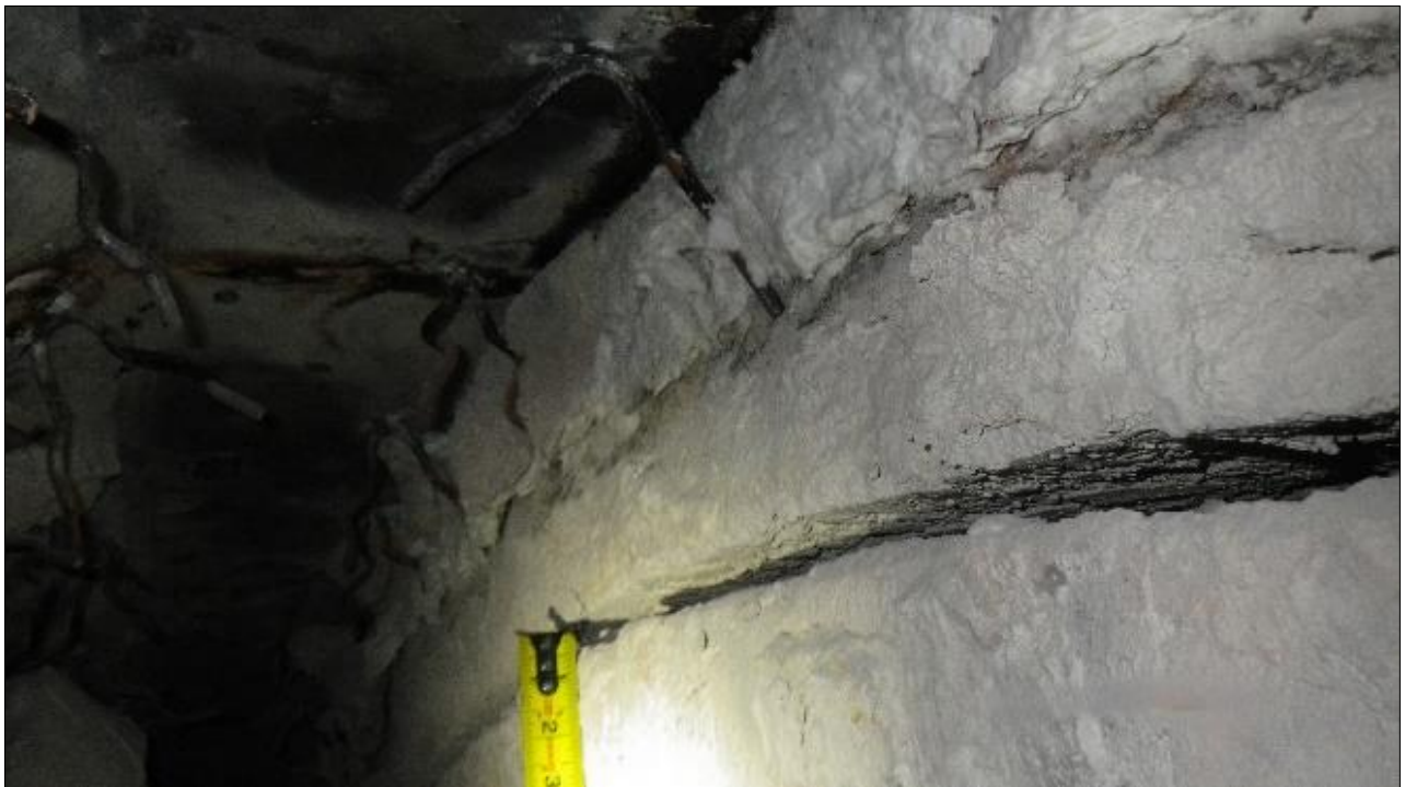
Figure 8: Thermal reactor hot face bricks along top center have sagged downward resulting in an open gap between hot face and backup layer.
