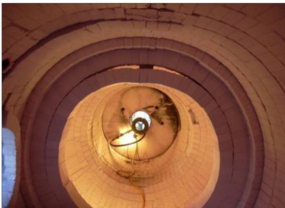
Figure 6: Thermal reactor choke ring with bricks above centerline flattening
